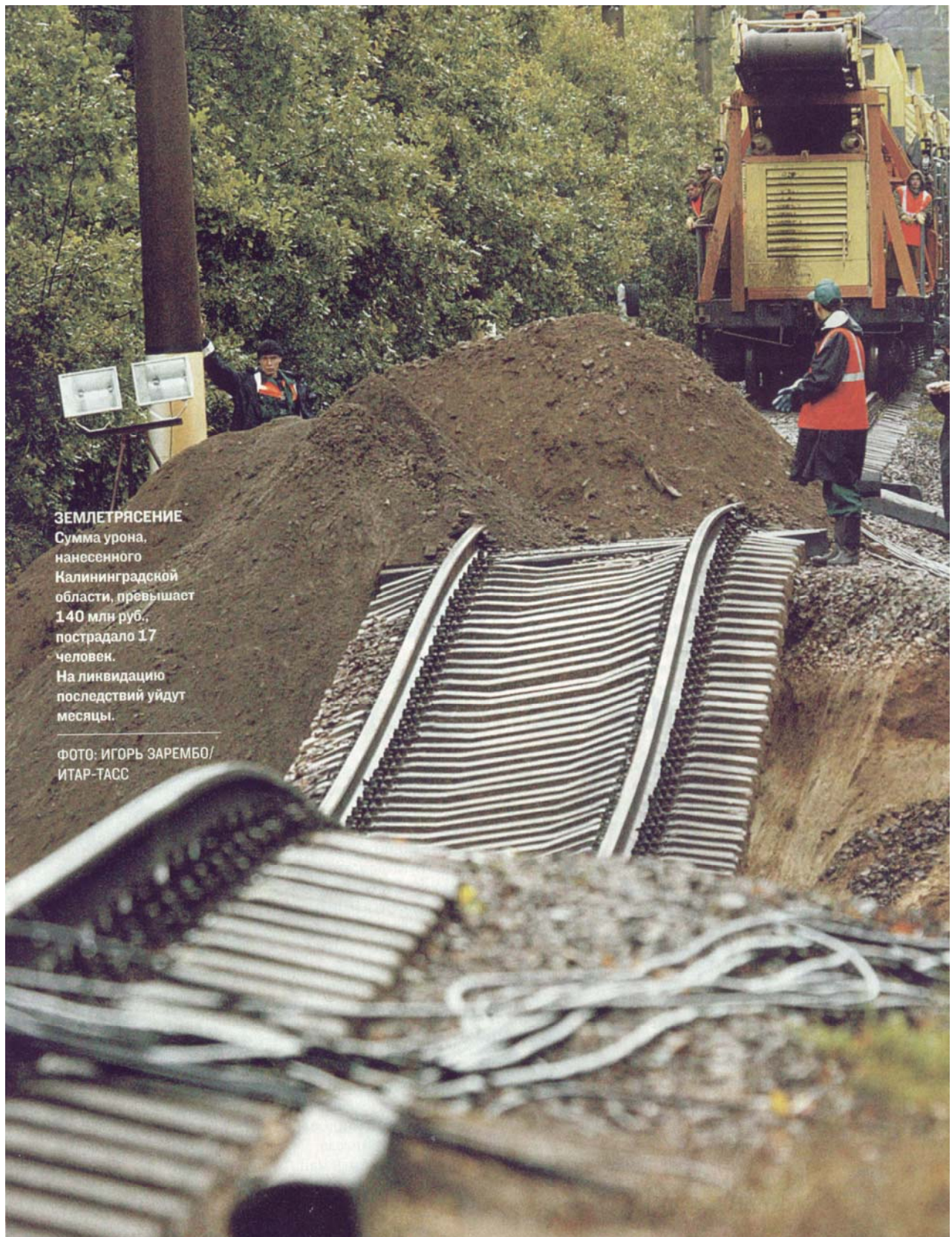
Fig. 1.2 The rail deformation. Zarembo from the newspaper “Komsomolskaya Pravda v Kaliningrade”.
