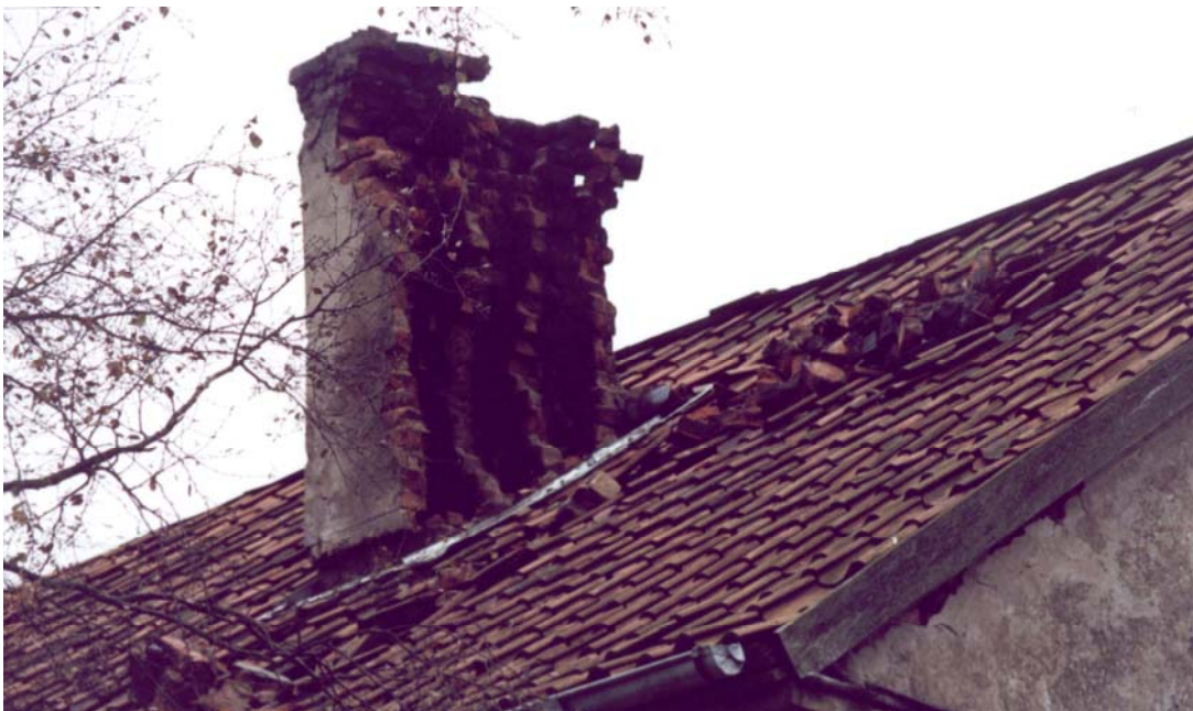
Fig. 1. 9 The damage of chimney. The bricks are thrown aside on distance larger than chimney height.
