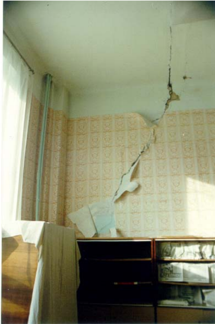
Fig. 1.5 The Children orthopedic sanatorium (3-storey brick building) in Pervomaisky town, first floor. The crack crossed inside wall through the entire three storeys diagonally.
