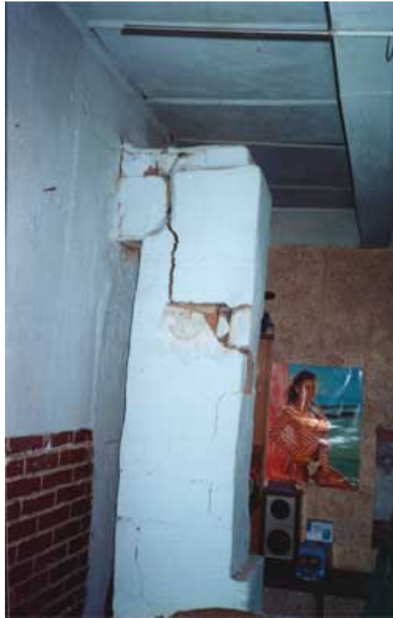
Fig. 1.8 The damage of oven.
