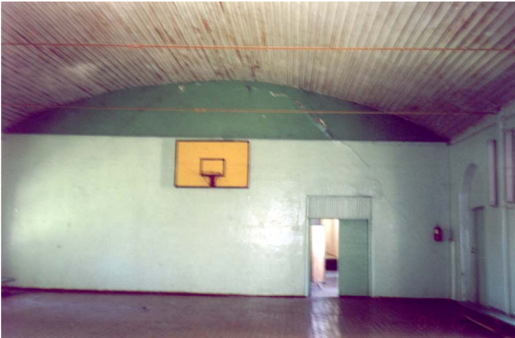
Fig. 1.6 The wall crack in the gymnastic hall on second floor of school in Primor'e town.
