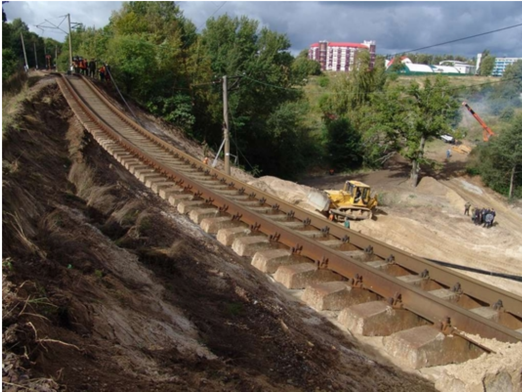
Fig. 1.3 The railway embankment sliding near Svetlogorsk town. The ground mass slid to sea side and railway was hanging on 15 meters high. This point is about 50 m apart from the place shown on Fig. 1.2. Photo I. Zarembo.
